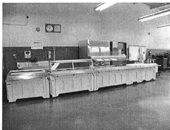
Unused Cafeteria Serving Area
