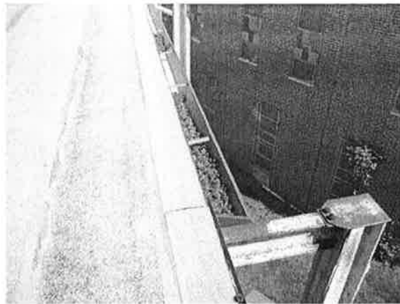
Roof and Gutters of 1970 Bridge
