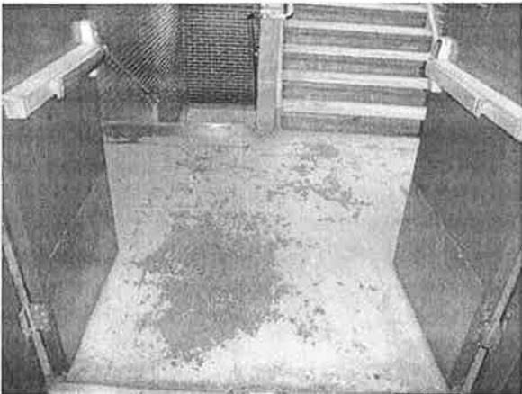
Painted Concrete Floor of Stairwell
