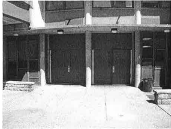
Exterior Doors to Gym/Annex Main Lobby
