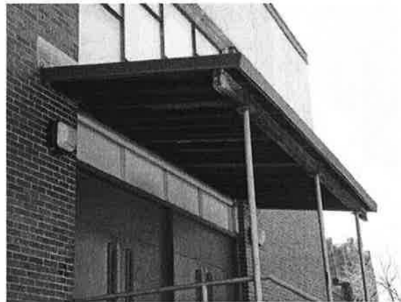
Metal Awning over Gymnasium Entrance/Exit
