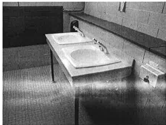
Typical Student Lavatories
