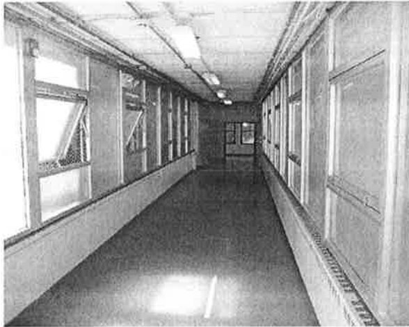
Interior of 1959 Bridge
