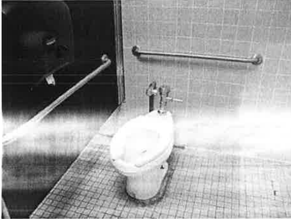
Typical Student Accessible Toilet and Stall
