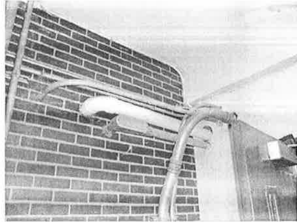
Conduit Penetrations through Stairwell
