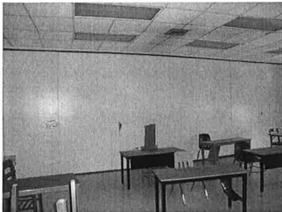
Movable Partition Wall - Vocational Classroom
