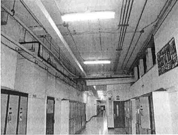
Basement Hallway with Open Ceiling
