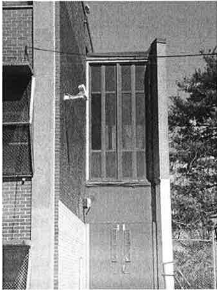
Annex Stair Tower
