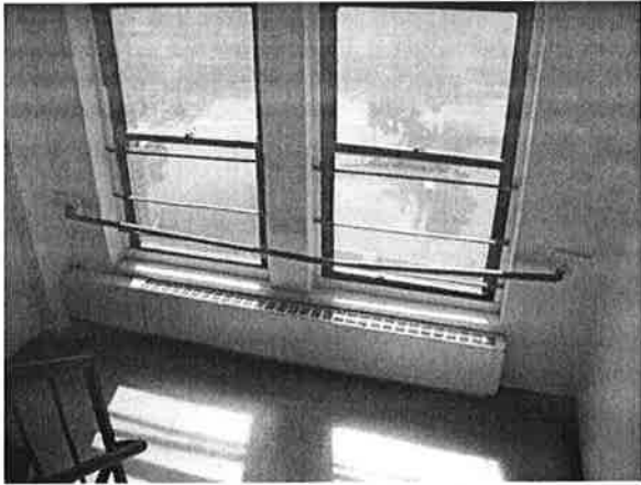
Typical Stairwell Corridor
