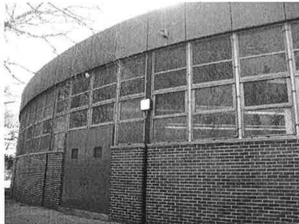
Typical Exterior of Vocational Wing
