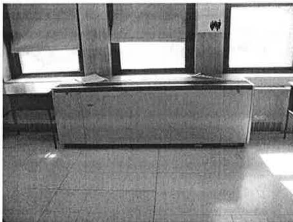
Typical Classroom UV
