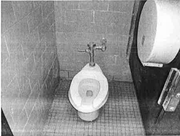
Typical Stall in Locker Room Toilet Room
