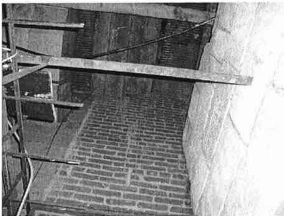
Interior Structural View Looking Up
