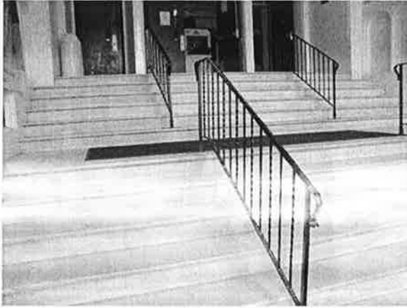
Interior of Main Entrance
