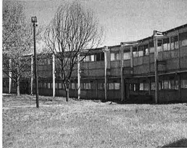
1970 Bridge – Parking Lot Side
