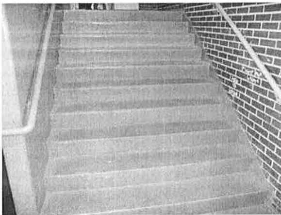
Concrete Steps in Annex Stairwell
