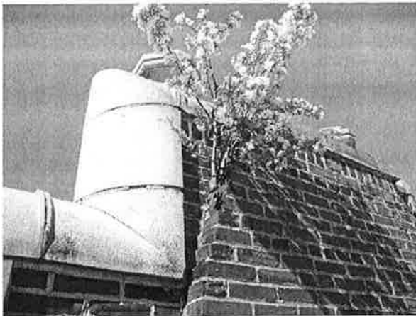
Parapet wall with Vegetation (common)
