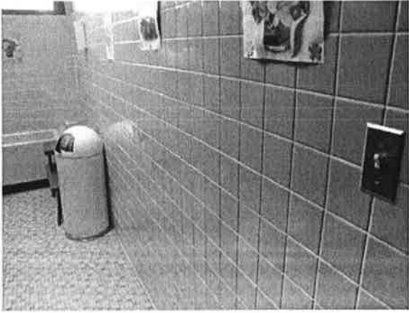
Typical Toilet room Wall Finish
