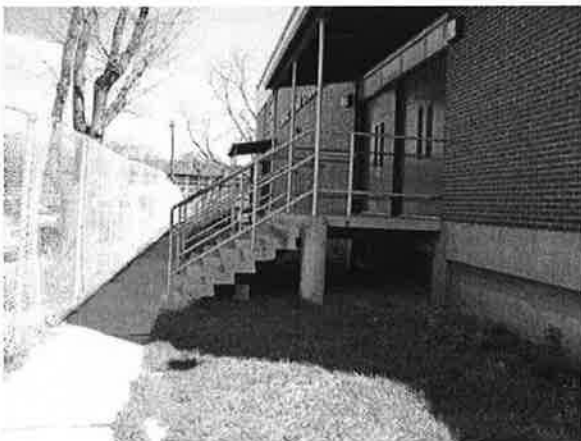
Gymnasium Entrance/Exit to Parking Lot
