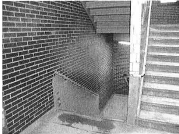
Typical Stairwell Corridor in Annex
