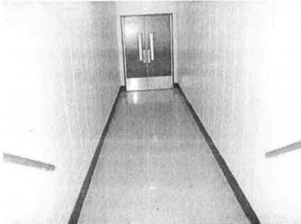
Stairwell Ceiling and Floor Finish
