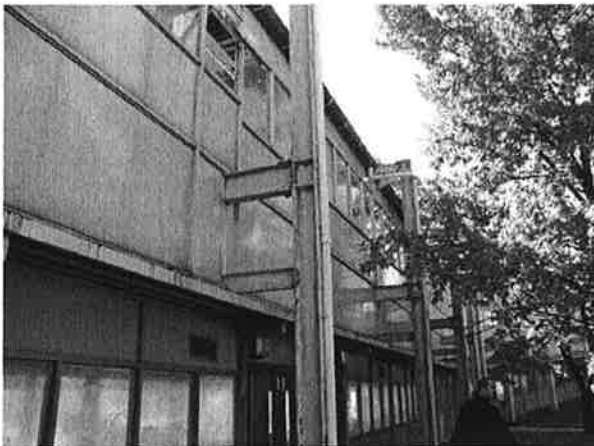
Steel Column Supports for 1970 Bridge
