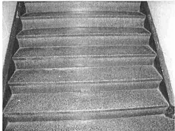
Terrazzo Stairwell in Vocational Wing
