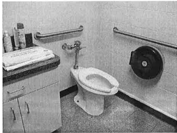
Typical Staff Toilet room
